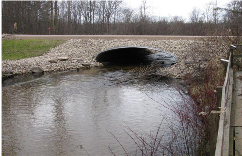
Road/stream crossing at 21 st Road – replaced in 2010.
